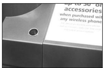
Step 1: The DC power outlets were not hooked up by the installers when the Verizon Wireless store was installed. You will need to run power to this outlet.
